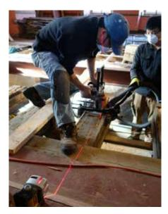
Routing out slots in old timbers using a precision guided electric chain router.
