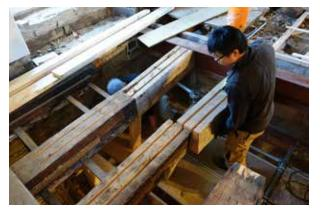
New and old timber sections prepared for insertion of reinforcing steel plates.
